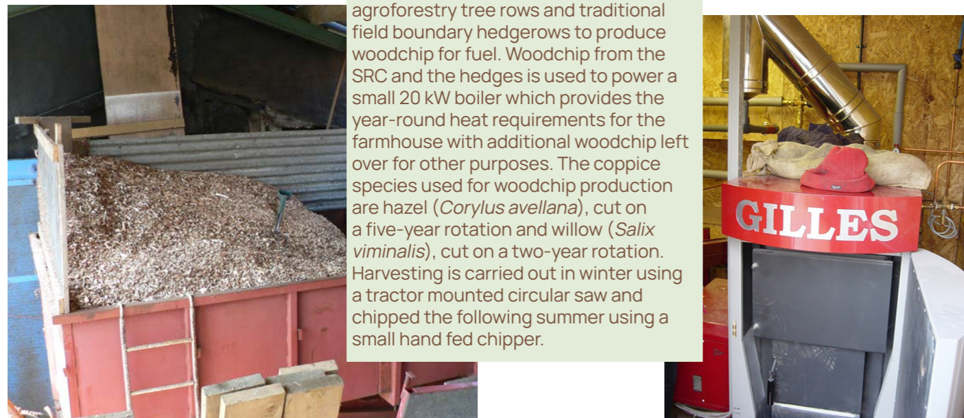
From field to boiler. Willow harvested, dried and chipped to feed into a woodchip boiler that heats the farmhouse.
