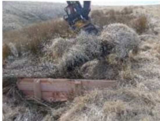
Grip blocking of drainage channels
