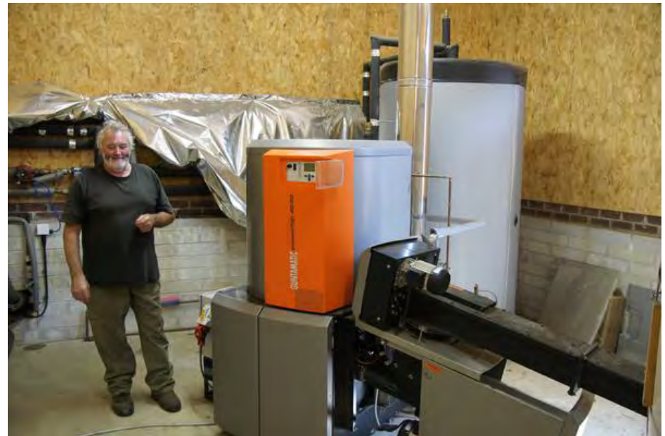
35 KW boiler, Lewmoor Farm
