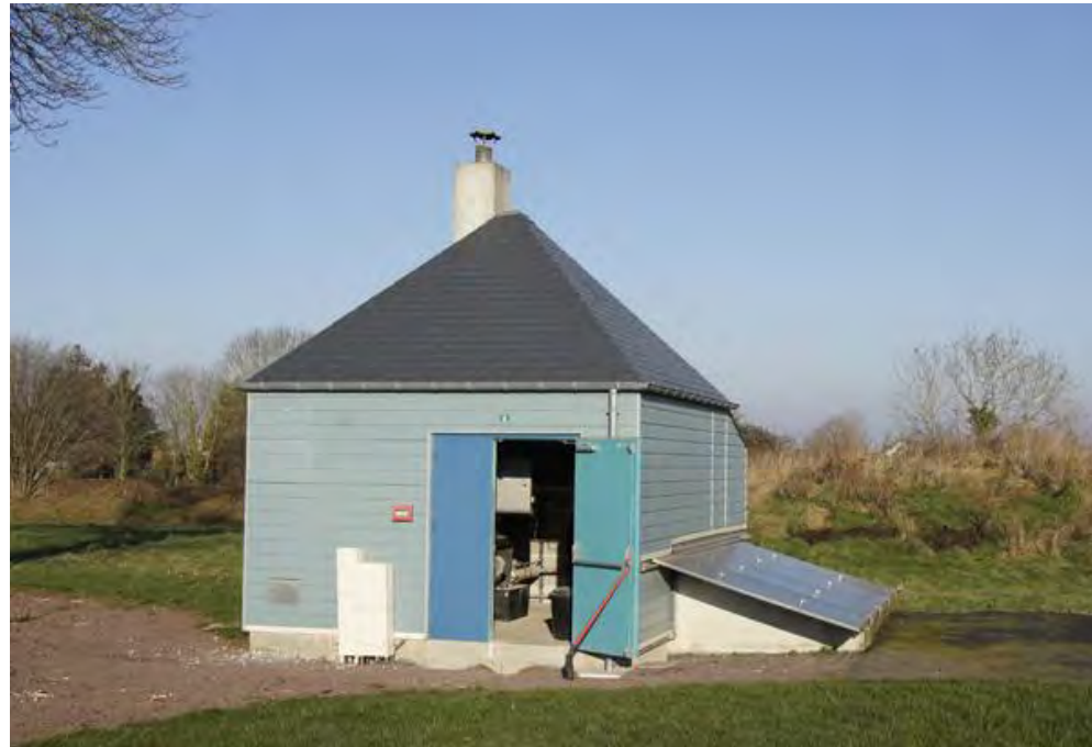
Community housing woodchip boiler at Samson-de-Bonfosse
