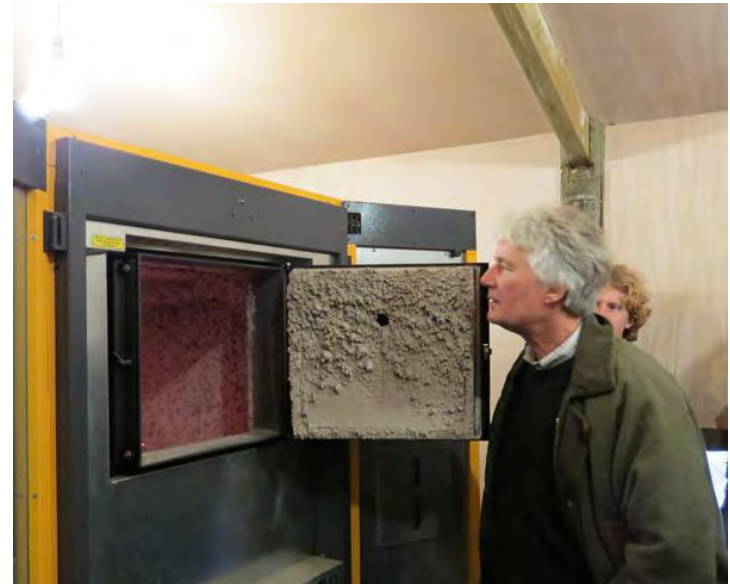
200KW woodchip boiler for 9 houses, Whitemoor Farm
